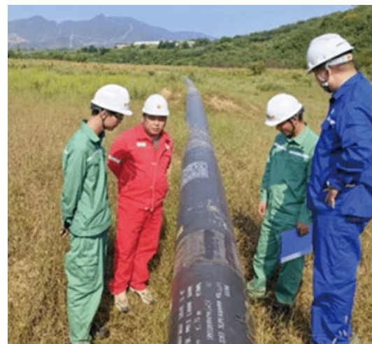
Luquan-Jingxing Gas Pipeline Project
