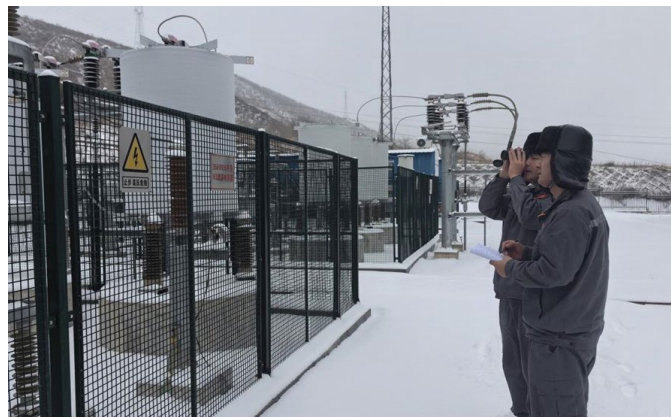
Caofeidian Suntien Liquefied Natural Gas's On-Site Inspection
